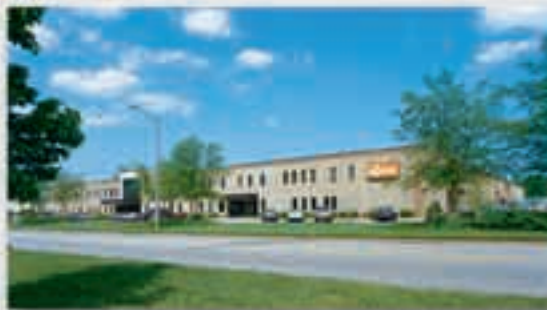
Manufacturing and Service Center Headquarters - Virginia Beach, Virginia Phone 757-463-7800
