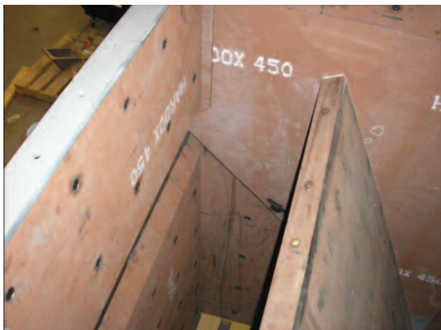
Abrasion-resistant steel liner
